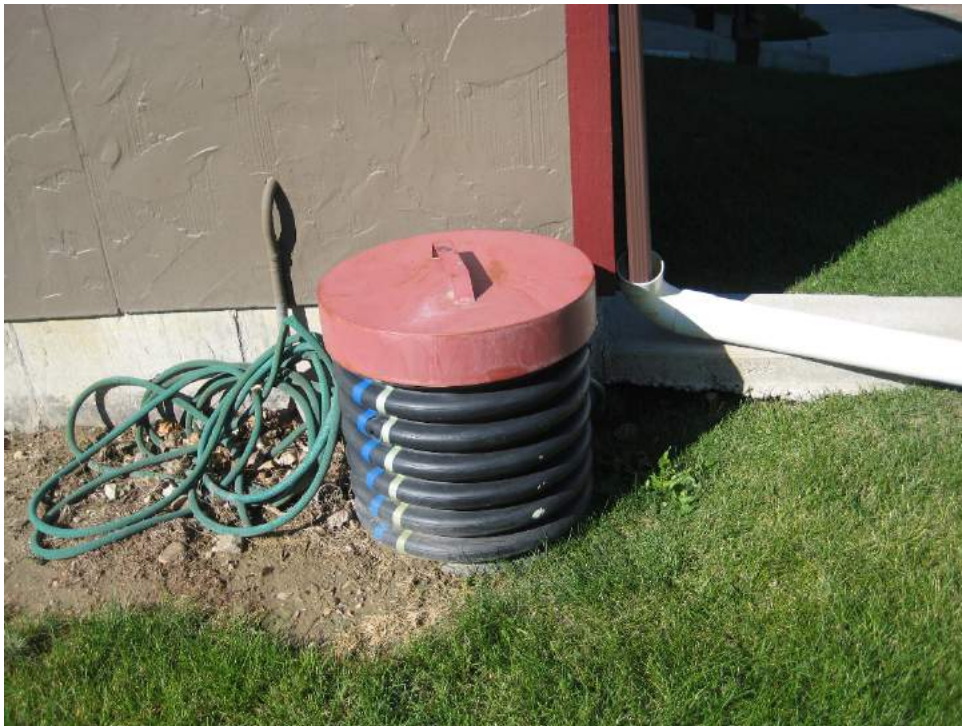
Photo 6. Part of the drainage system used to address the flooding in the easternmost apartments.
